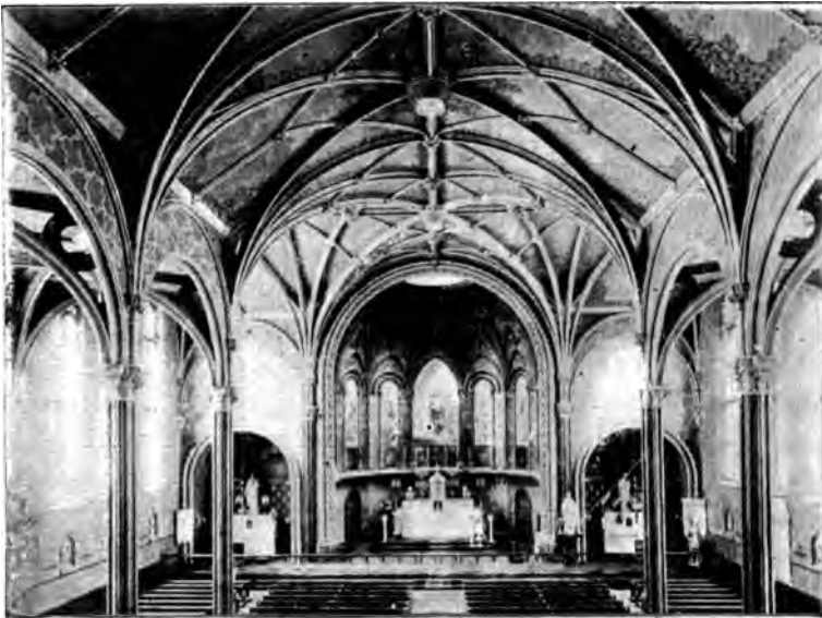
INTERIOR OF ST. JOHN'S, UTICA, THIRD CHURCH.
